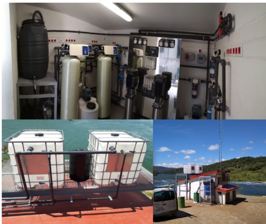
Fig. 4. Above: Picture of the water treatment plant. Below left: 1 m 3 water storage tanks for rejected and pure water. Below right: Arrocampo water discharge monitoring station.
