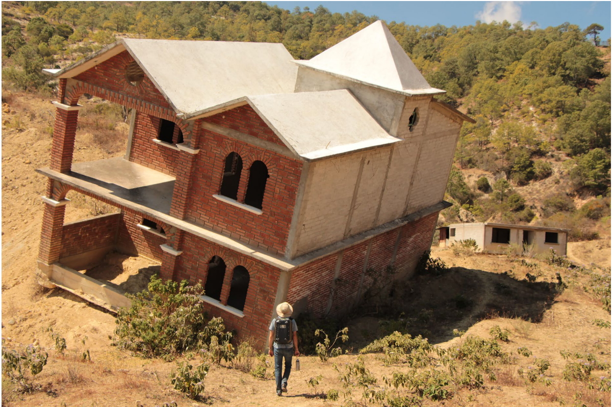
Fig. 6 An image of one of the houses displaced more than 200 meters from where it was originally built. February 2021
