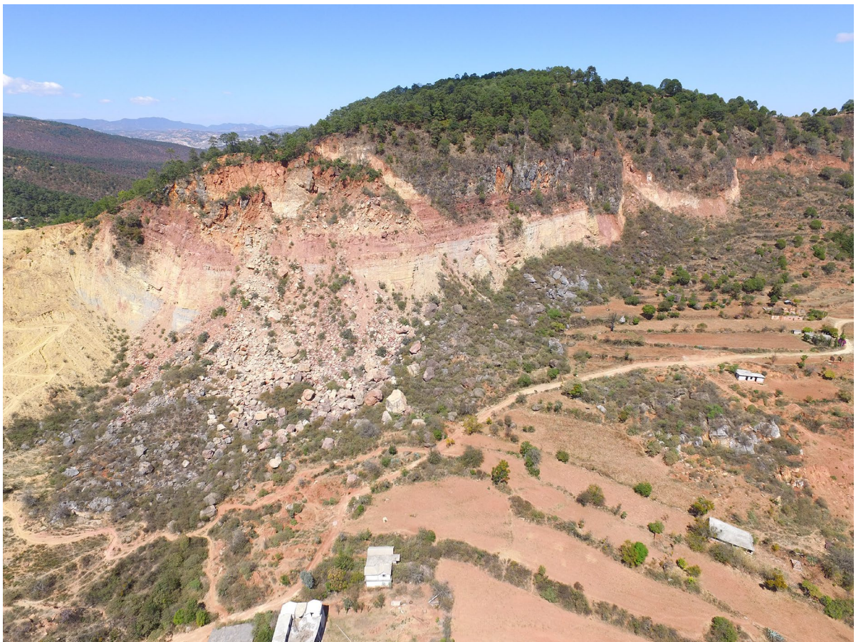
Fig. 1 Rupture zone located on the northern flank beneath Peña Colorada hill, February 2021
